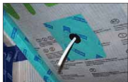
Use of rubber gasket to seal a penetration of the airtight membrane. Source: MosArt Architecture
