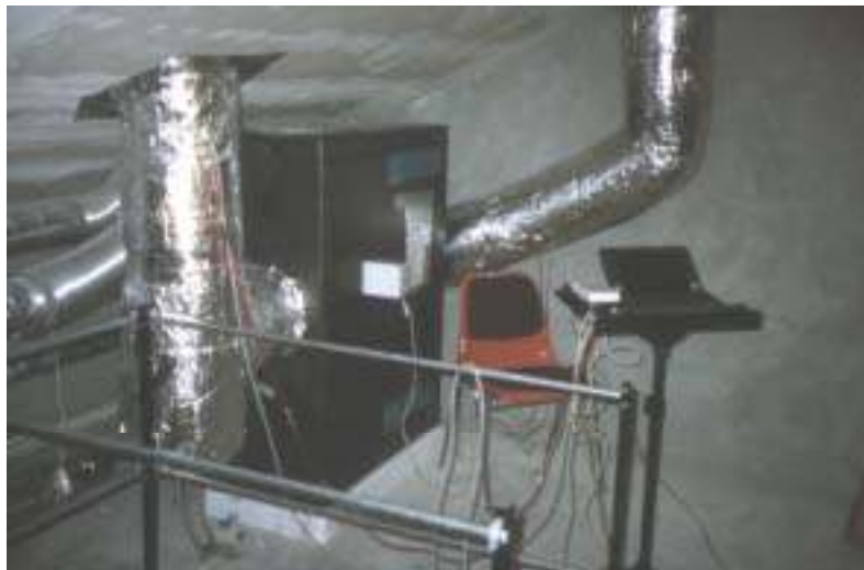
Figure 36: Measurement technology set-up for the balance calibration of the heat recovery system in the building services floor of one of the Passive Houses. With the use of pressure measurement, the volume flows at the differential pressure sensors in the in- (right) and outflow (left) ducts were determined and evaluated. The outputs of both ventilators were individually set-up with the manufacturer's operating device.
