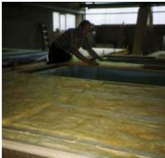
Figure 29: The insulation must lie loose and slightly inflated within the element, so that no cavities are formed later
