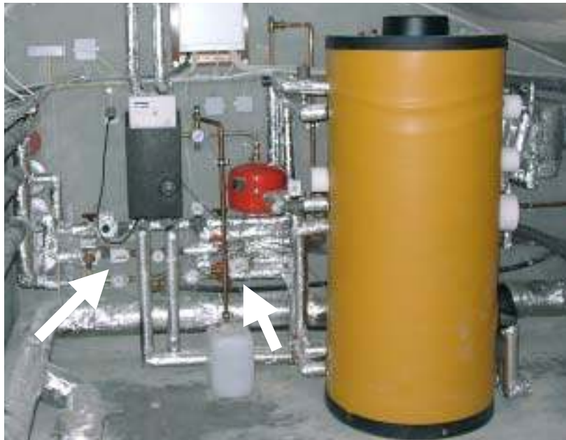
Figure 41: Installation wall on the building services floor with water storage tank. The two heat quantity meters are marked with arrows.
