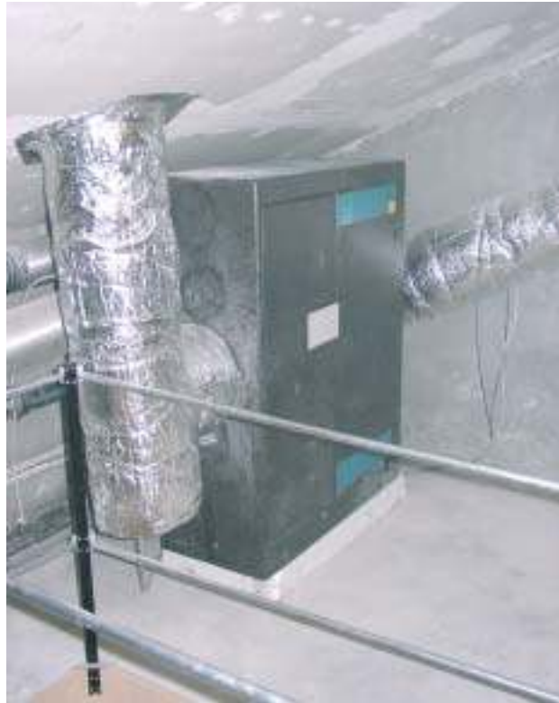
Figure 21: Ventilation unit with heat exchanger in the building services floor of a Hannover-Kronsberg Passive House. In the background is the fresh air duct with defrost heater and in the foreground is the exhaust air pipe (both insulated with mineral wool, aluminium laminated)
