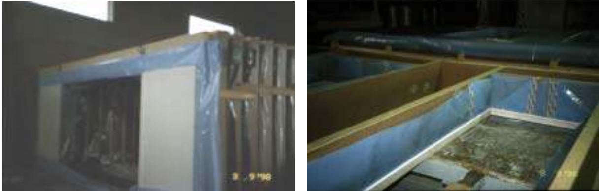
Figure 30 (left): Facade element window opening. The airtight foil joints are carefully glued, the overhanging foil is there to allow for an airtight seal with the next elements
