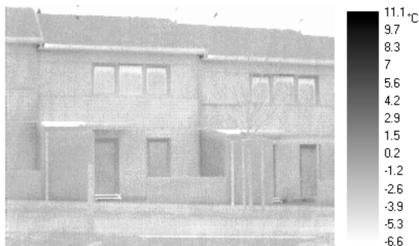
Figure 34: Outdoor thermograph of a section of the houses in row 9 (north side). The area under the roof overhang and under the canopy over the main door seem warmer, since these areas are „covered“ from radiation into the cold night sky. Otherwise, the facades show continuous low temperature of around -4\text{ °C} .
