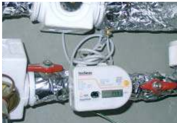
Figure 42: Total heat quantity meter on the installation wall of the building services floor. The cable leads to the temperature sensor (Pt 500) in the supply pipe.
