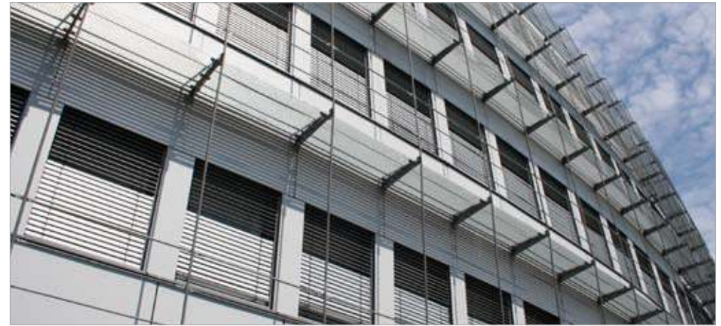
Plate 2.4.1 The shading blinds on this office building, when fully extended, remain open at the top to allow daylight deep into the office but are closed at the bottom to reduce glare at desk level
