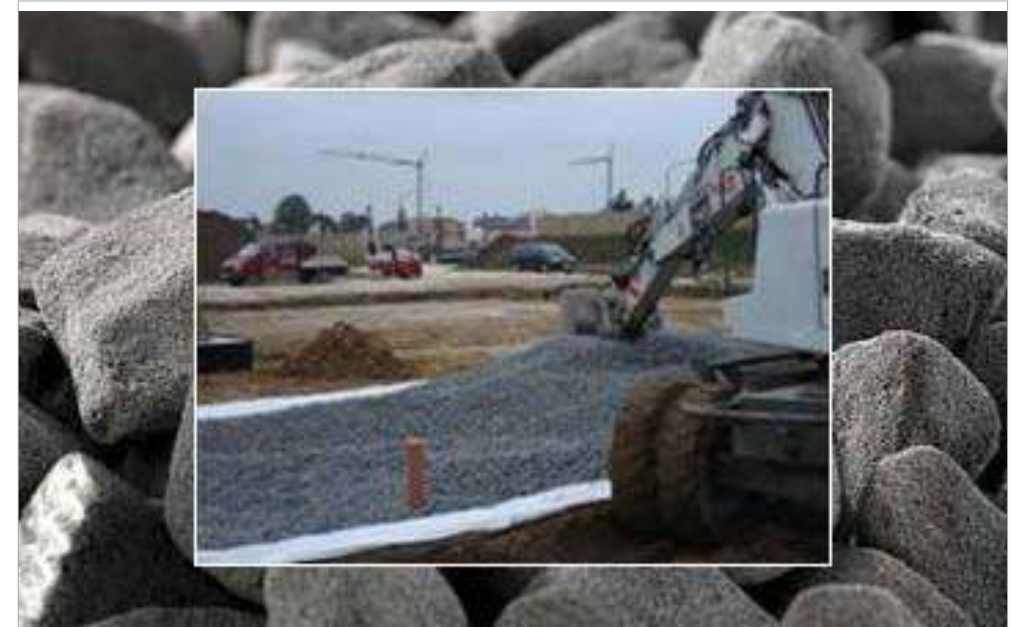
Plate 2.1.1.1.9 Structural foamglass insulation for use under floor slabs
