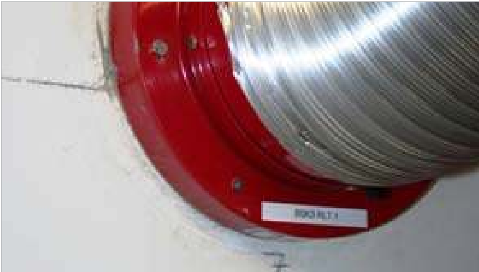
Plate 3.4.2.4 Fire compartmentalisation devices in centralised ventilation systems
