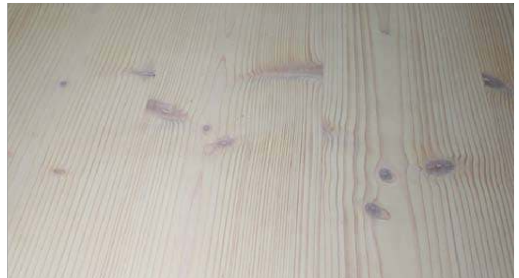
Plate 3.3.3.3 The internal wooden finish of this gymnasium was finished with a white wash to reflect more natural light within the building
