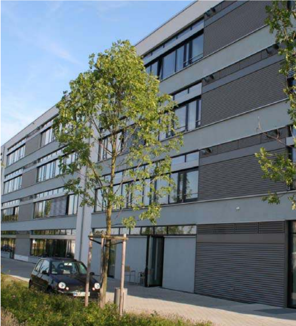
Plate 3.1.1.1 The proportion of glazing in office projects is optimised to create a balance between maximising solar gains in winter and minimising risk of overheating in summer
