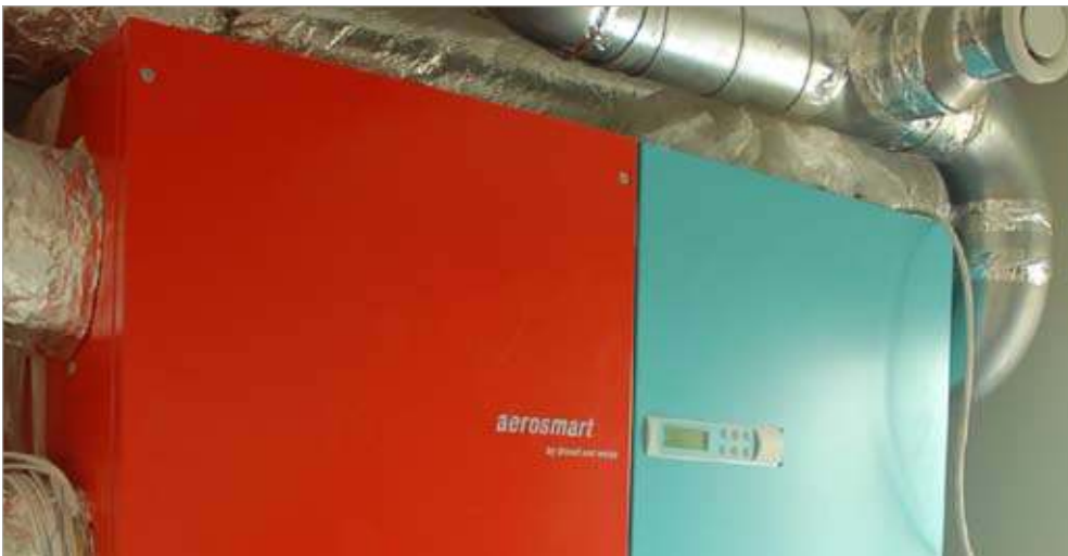
Plate 3.4.2.1 Compact units such as that depicted above are well suited to apartment projects where space might be limited for more bulky plant
