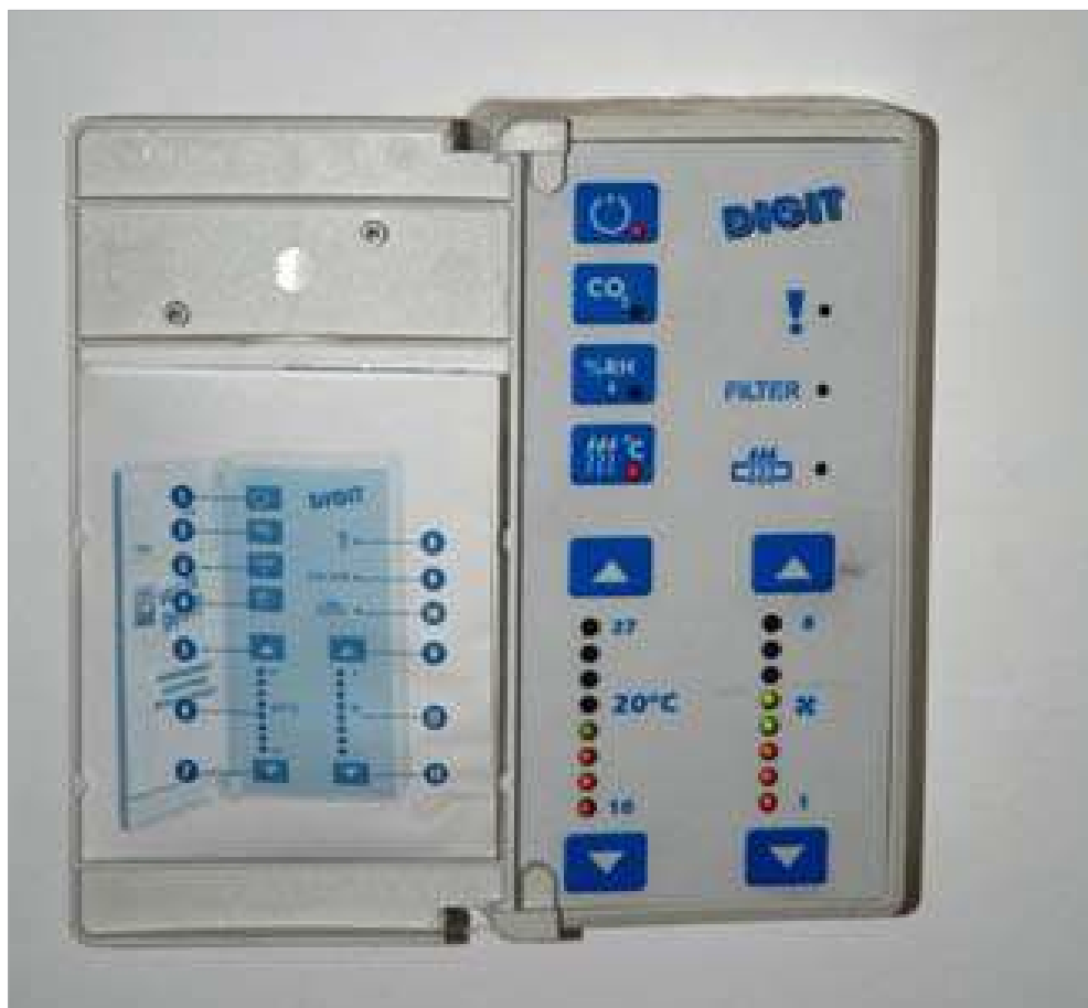
Plate 3.4.4.1 Typical control unit for MHRV in an apartment which will inform the home owner when the filter needs to be replaced
