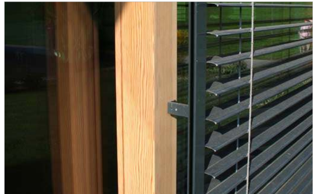
Plate 2.4.2(a) and (b) Retractable shading can be fitted to the external facade and controlled either manually or automatically
