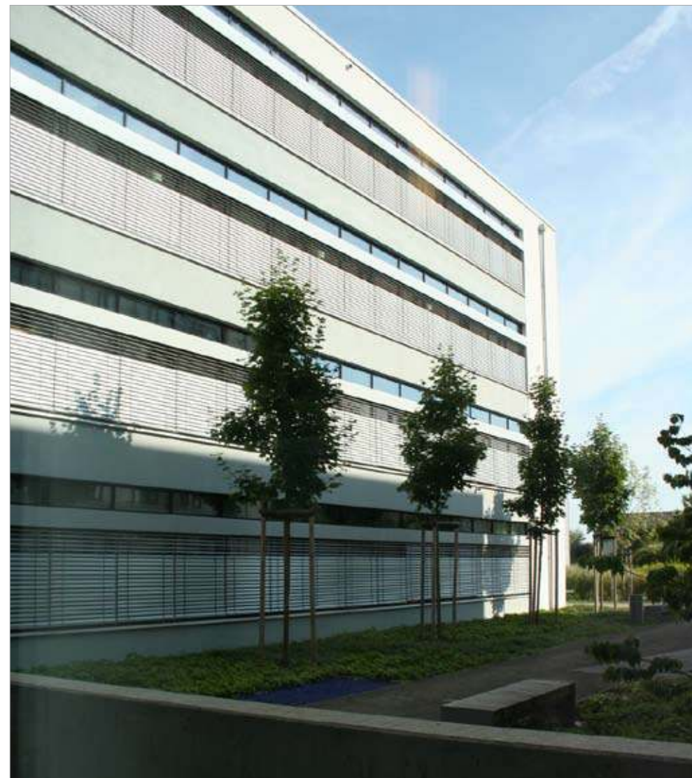
Plate 1.2.2. Shading devices are generally required to reduce overheating
