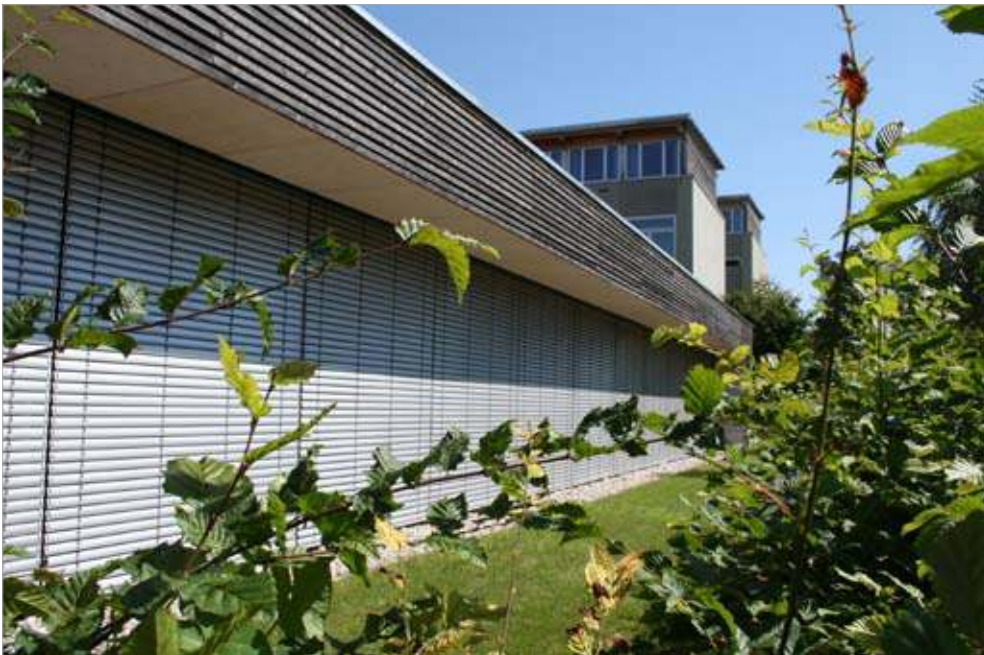
Plate 3.3.3.1(a) and Plate 3.3.3.1(b) External shading can be extended or retracted to control glare for sports activities and to minimise risk of overheating
