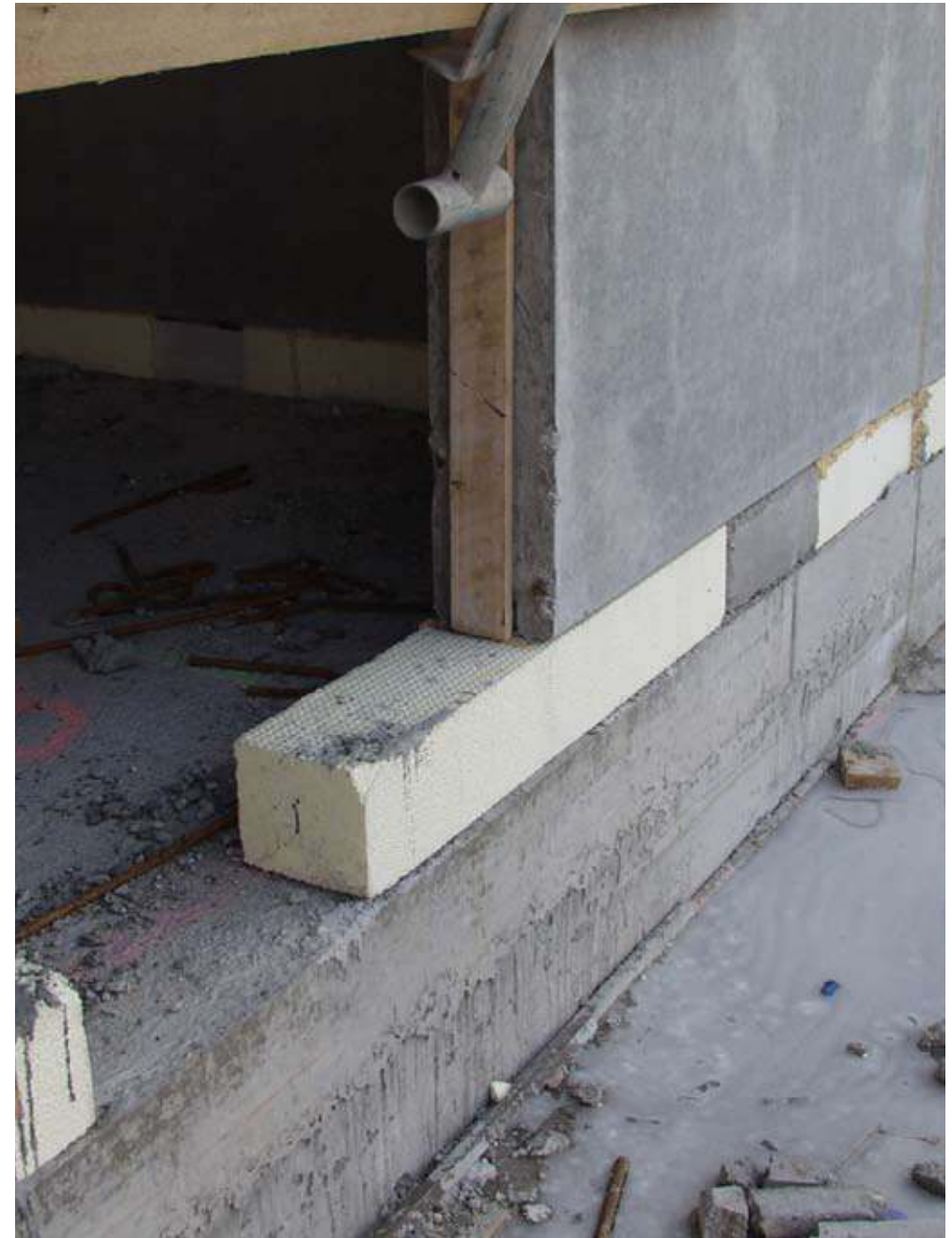
Plate 2.1.1.1.5 Hybrid thermal break used in masonry multi storey apartment projects.
