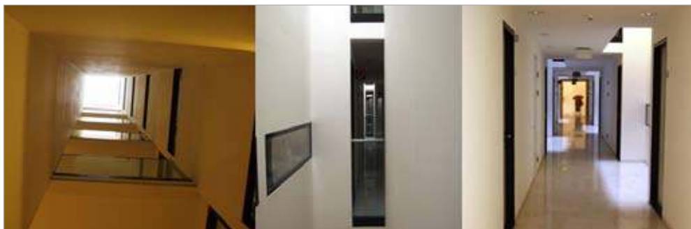
Plates 3.4.1.1(a), (b) and (c) Light shafts in apartment blocks can be designed to provide daylighting for both semi-private circulation space as well as private living space
