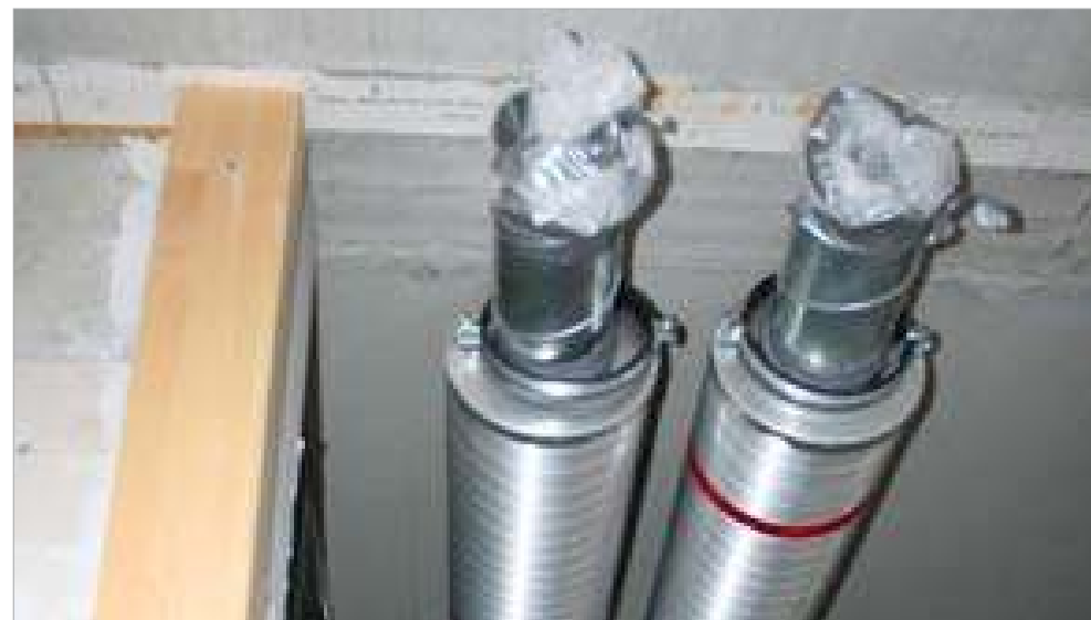
Plate 3.4.2.2 Decentralised MHRV system in apartment ceiling void during construction
