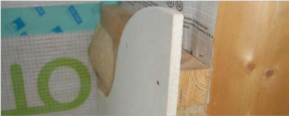
Plate 2.1.3.5 Providing an internal service cavity will ensure protection of the air-tightness barrier in timber frame construction
