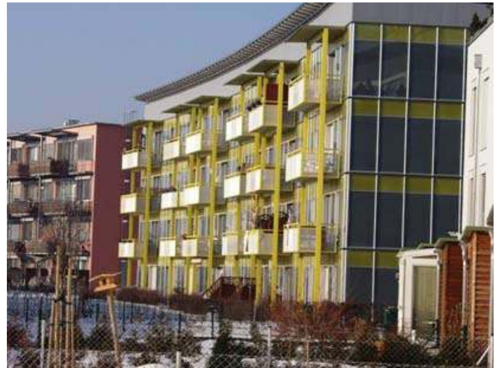
Plates 3.4.3.1 Balconies often serve dual purpose in providing both access to external space as well as providing shading to south-facing windows
