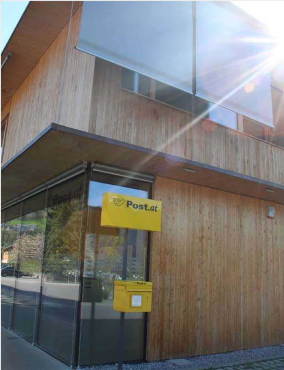
Plate 2.4.3 These retractable opaque blinds are restrained by guide wires but would have to be carefully considered in windy or exposed locations
