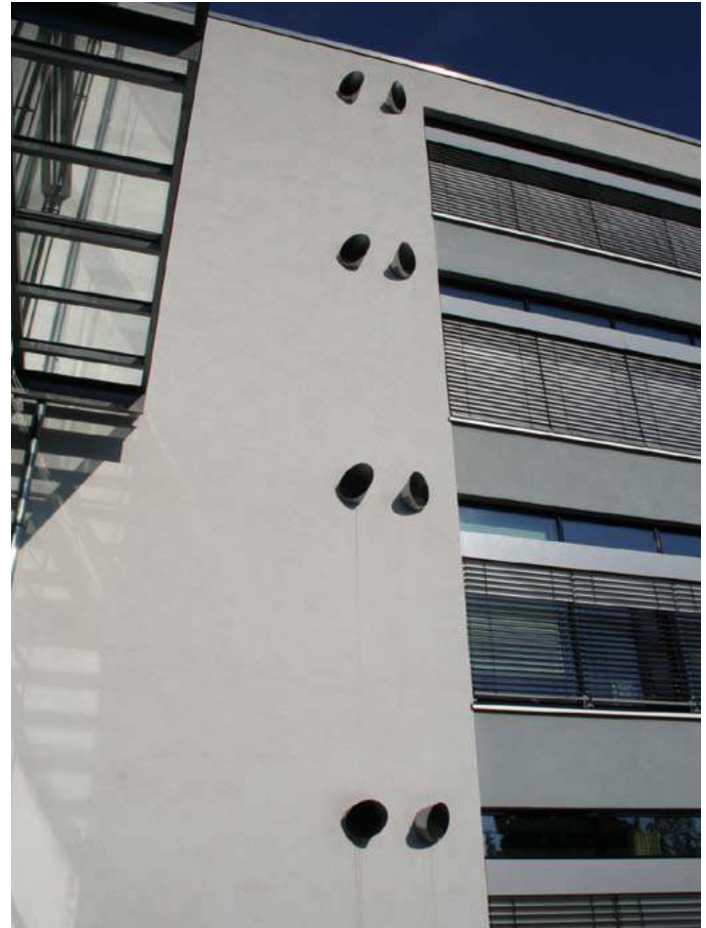
Plate 3.1.2.1 The decentralised ventilation system provides flexibility of internal layout options
