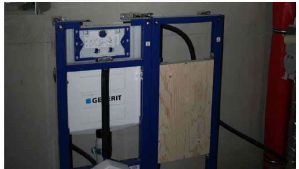
Plate 2.1.3.4 Note how the rear of this fixing for wall mounted services was plastered in advance of installation, ensuring air-tightness
