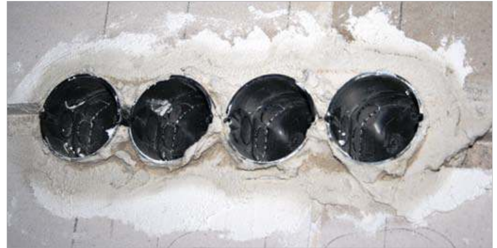
Plate 2.1.3.3 In masonry construction where there is no service cavity, it is important to make any penetrations for services as airtight as possible, in the above case used by bedding the fixings into wet plaster
