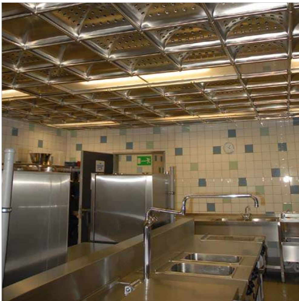
Plate 1.2.5 Commercial kitchens present a challenge in terms of ventilation
