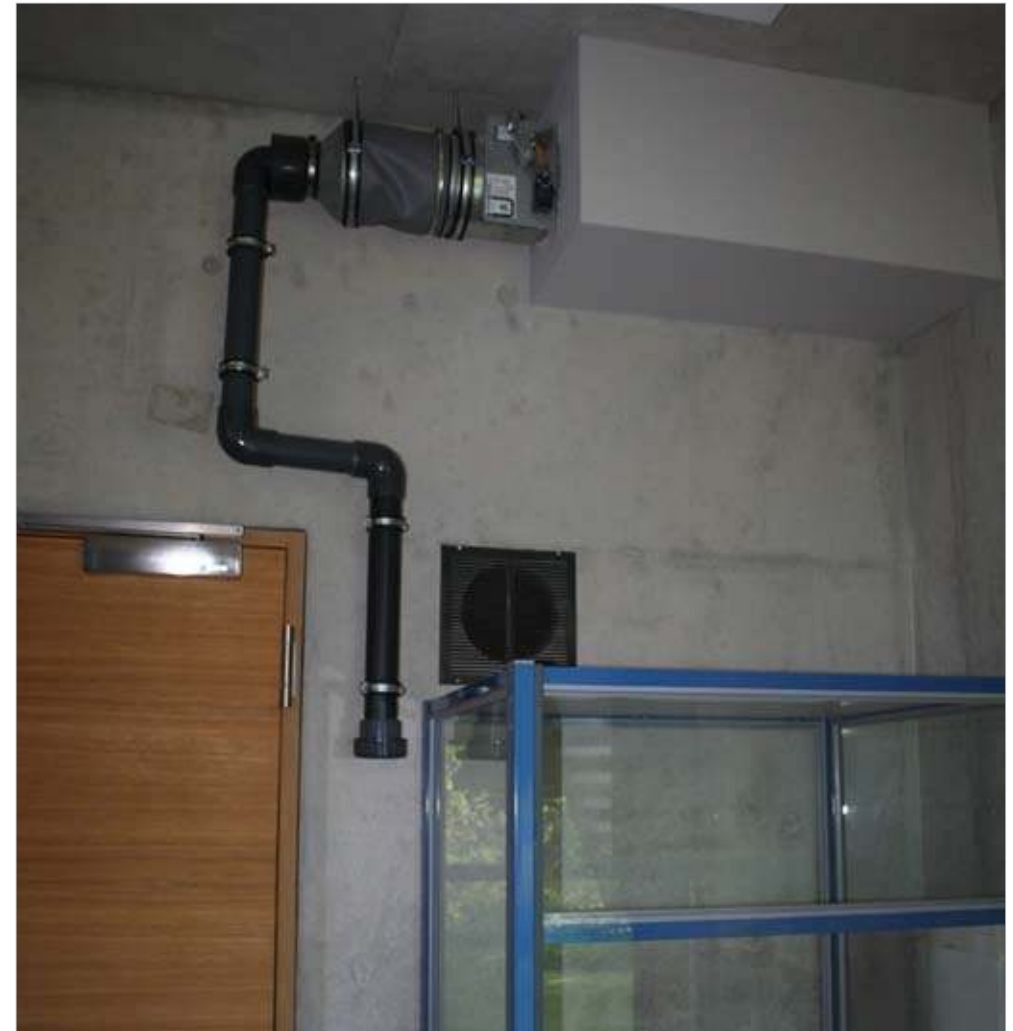
Plate 3.2.2.1 Fume cupboards in laboratories will need separate extract systems
