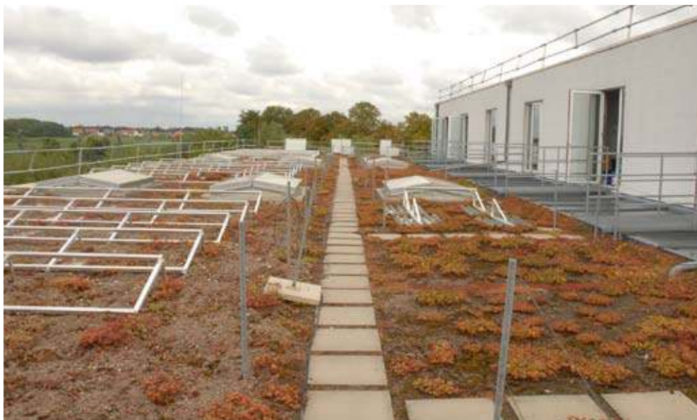
Plate 1.1.10 generally reducing cooling demands leaves roof space for renewable technology (in this case PV cells are being retrofitted to the roof of a commercial project)
