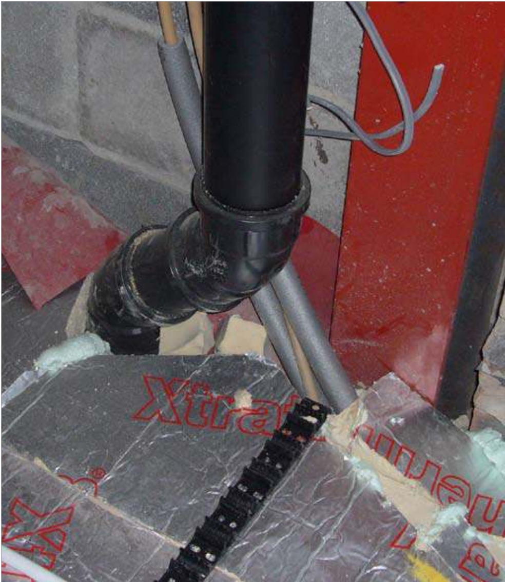
Plate 2.1.3.2 It would be impossible to make the above construction airtight – this is a result of poor planning
