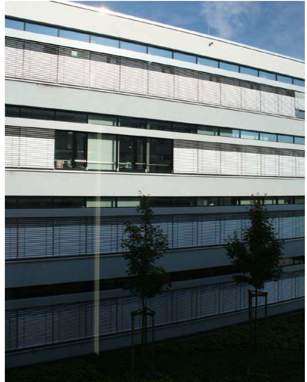
Plate 3.1.3.1 Shading mechanisms are most usually controlled by solar irradiation sensors as well as wind anemometers, the latter retracting the blinds if structural damage to the blinds is a risk.
