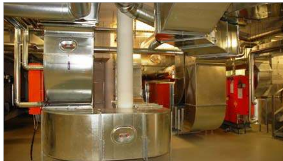
Plate 3.4.2.3 Bulky centralised MHRV systems require considerable floor space
