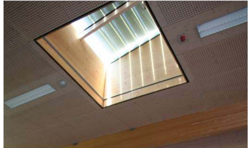
Plate 3.3.3.2 Natural daylighting can also be provided through energy efficient rooflights, coupled with bris-soleil to reduce overheating when the sun is high in the sky
