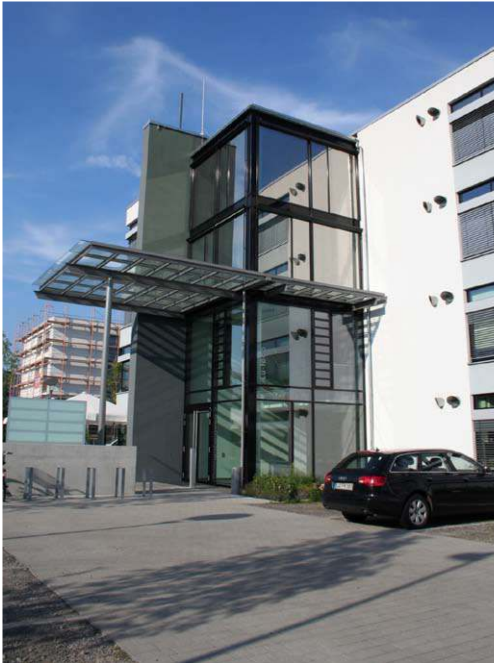
Plate 3.1.1.2 Entrance to the Luteco Offices in Ludwigshafen, Germany
