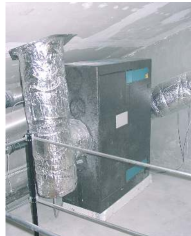
Figure 11 Insulation of ductwork, source: PHI
